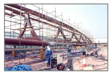
be as much as 40m (120ft) long, 4m (12ft) high and 2m (6ft) wide. Obviously, this is too large for the average hot-dip galvanising tank. The process is also transportable, so structural steelwork can also be sprayed on-site or repaired where on-site welding has removed the galvanising.
